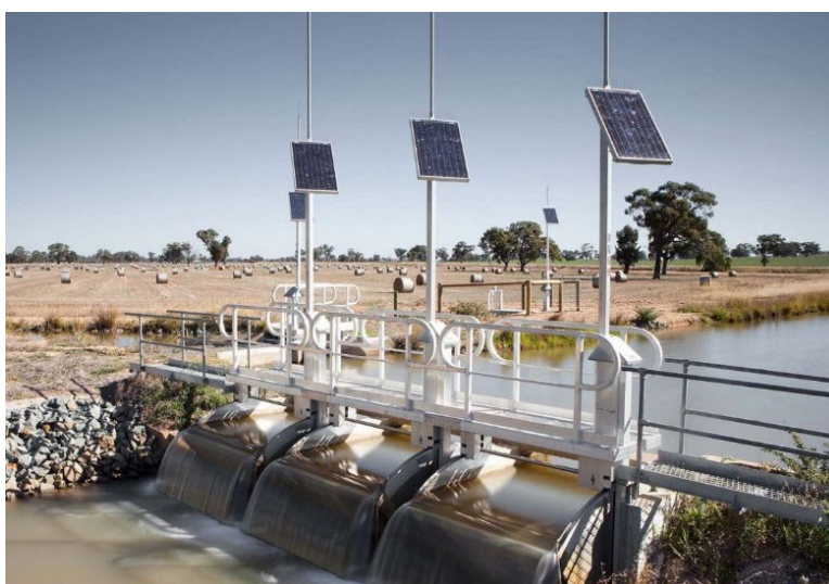
Figure 9.2 Rubicon Water's FlumeGates are a key component of the TCC solution
